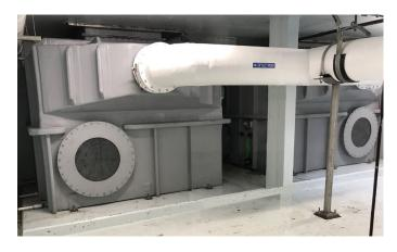
need for extensive customization. PureAir met this challenge by designing and constructing two Packed Bed System (PBS-709) units to treat a total max airflow of 7,500 C FM (1,875 CFM per unit) of foul air. Each unit was filled with CPS Blend chemisorbent media to ensure optimal performance.
