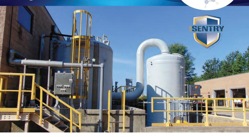
PureAir Filtration's Sentry<sup>™</sup> Emergency Gas Dry Scrubber is the best line of defense against toxic gas leaks at facilities that use gases that could be harmful to health and safety if released; such applications include chlorine tanks used at water treatment plants. With only one moving part, the Sentry<sup>™</sup> is safer, more reliable, and easier to operate than old fashioned wet scrubber systems, also requiring less maintenance and costs.
