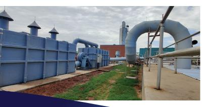
PureAir custom manufactured and engineered a Dual Train system with two VBS-720 scrubbers. The system was designed to capture the malodorous air through the bottom of the first unit as it passes through a media bed of Sulphasorb FeXL<sup>TM</sup>, then it moves through a header and into the blower of the bottom of the second unit where it encounters another media bed filled with Sulphasorb XL<sup>TM</sup>.
